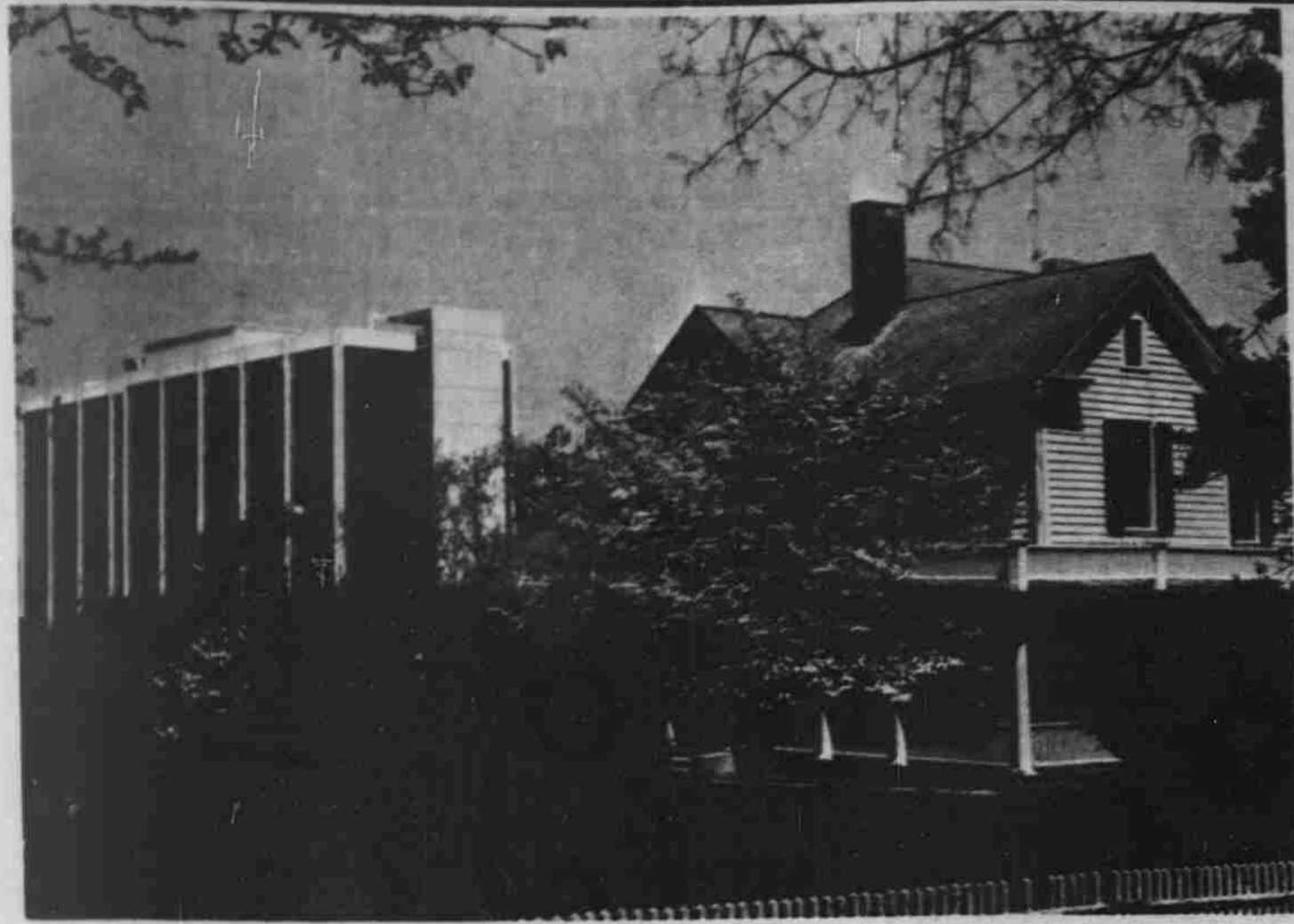
Granville Towers looms behind the 70-year-old Eubanks home ... part of the vanishing Chapel Hill, succumbing to age.
