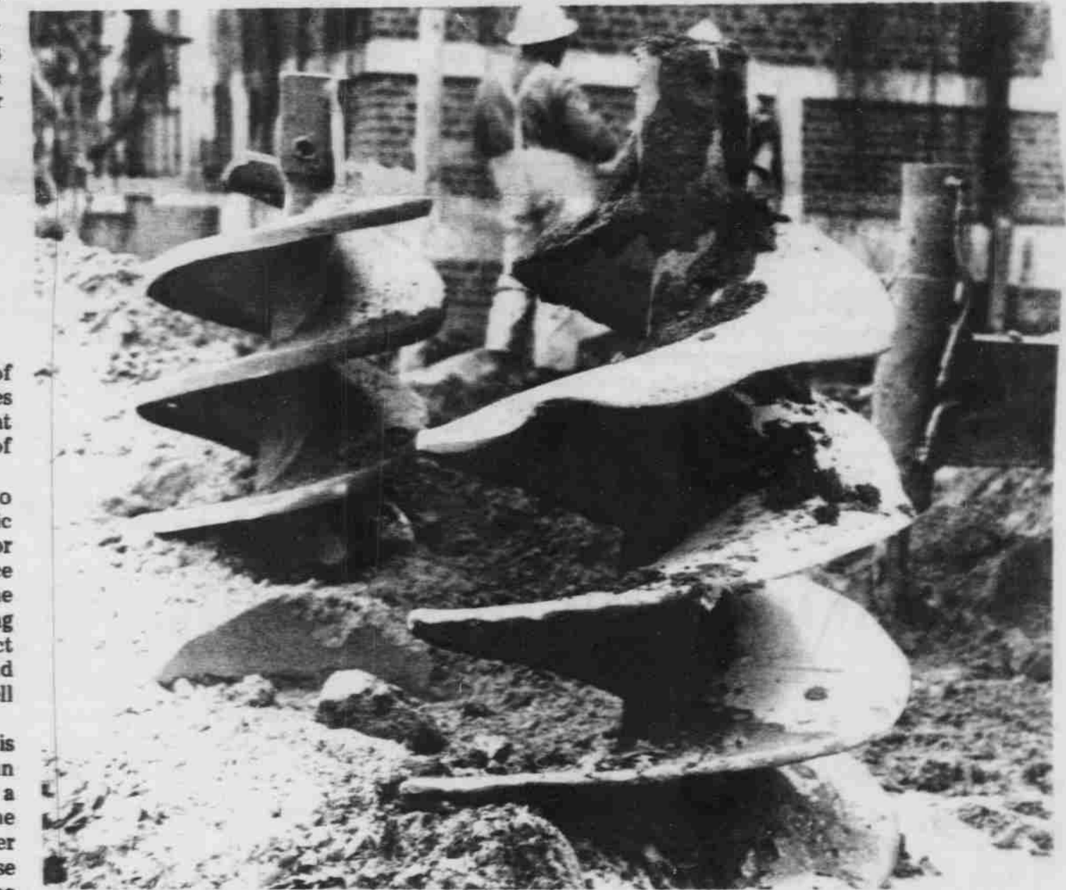
Drills Come Out Of The Ground At Bingham Construction Site
