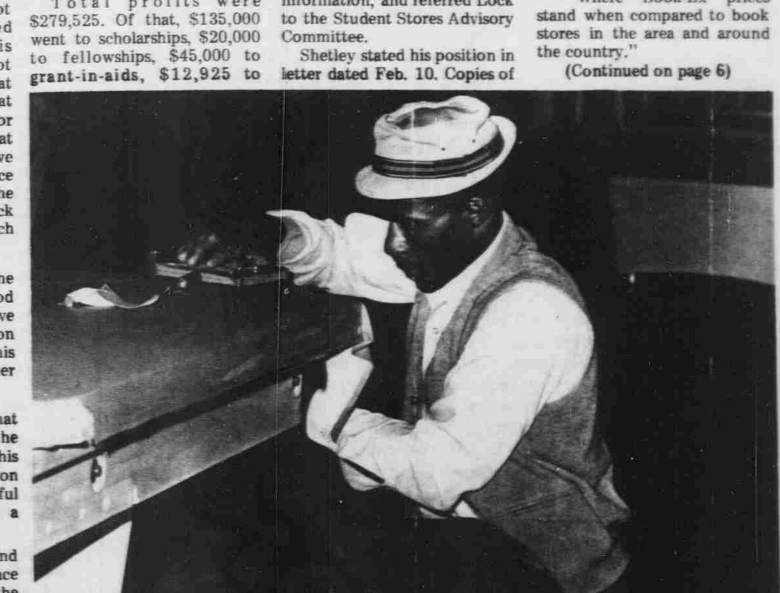
A Worker Installs The New Pool Tables ... In The Lower Level Of The New Student Union
