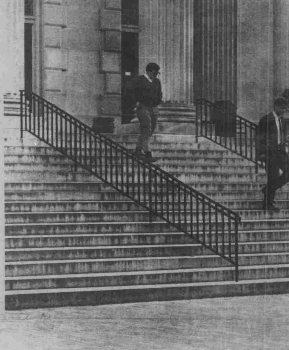
Wilson gets new railings
