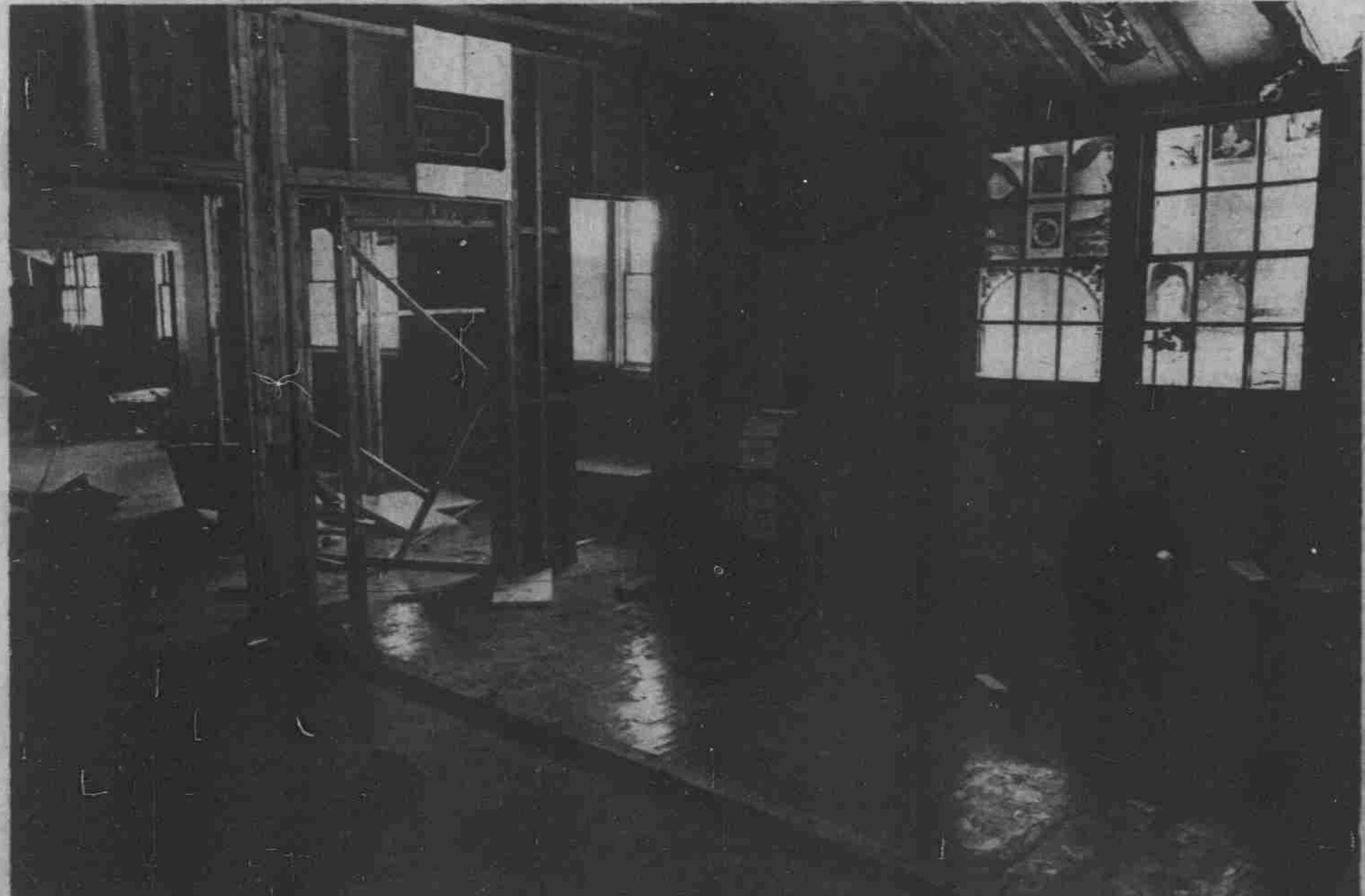
Bingham X, one of the old white buildings sitting adjacent to the Carolina Union parking lot, is scheduled for demolition in the near future. Currently the building is empty but not too long ago it was used by art students for a study.
