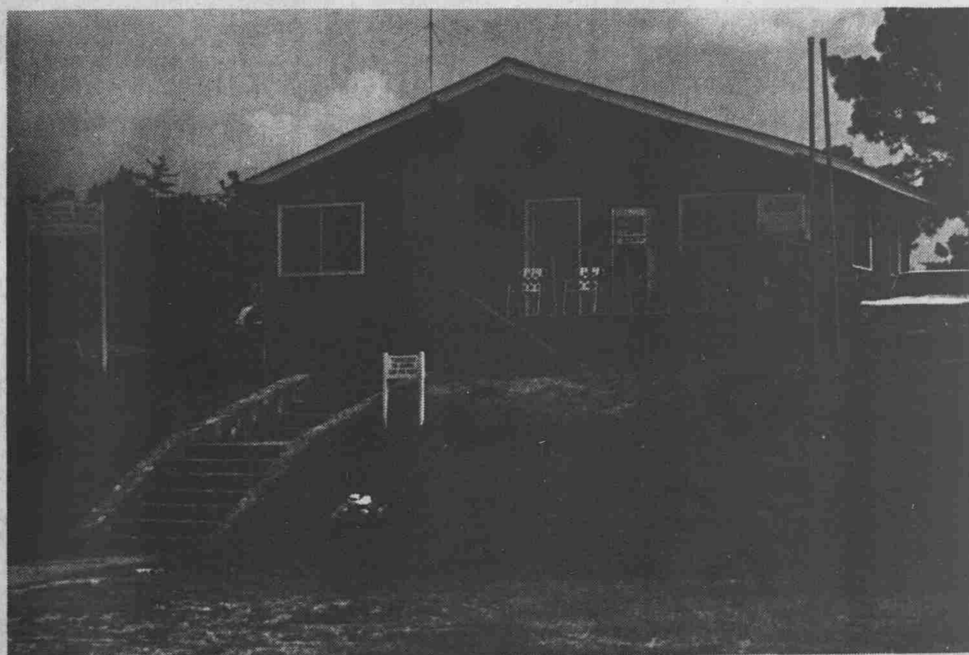
This is the terminal-lobby-administrative office of the University's Airport. It's a small-scale operation
