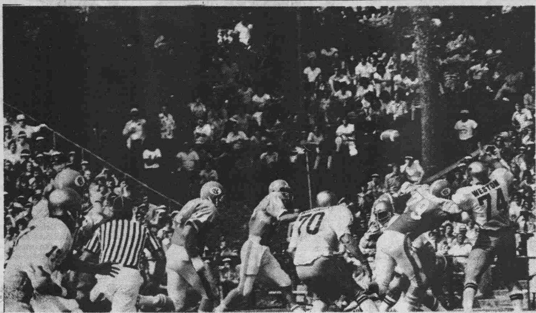
Work on the Kenan Stadium addition has been postponed until the end of fall, at which time the temporary bleachers (shown at left) will be replaced with permanent seats. Staff photo by Charles Hardy
