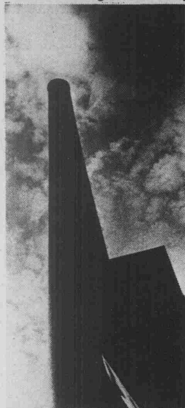
Power plant smokestack
