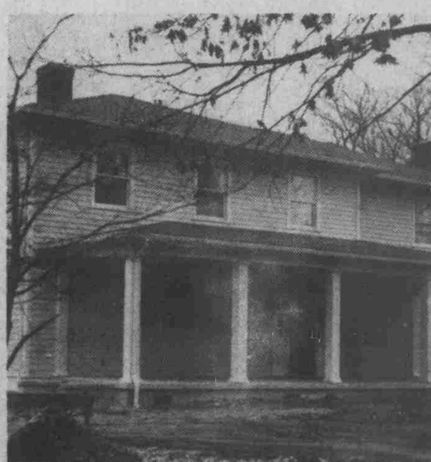
Zoning laws will help Greek house growth...Alpha Chi Omega house on Rosemary Street
