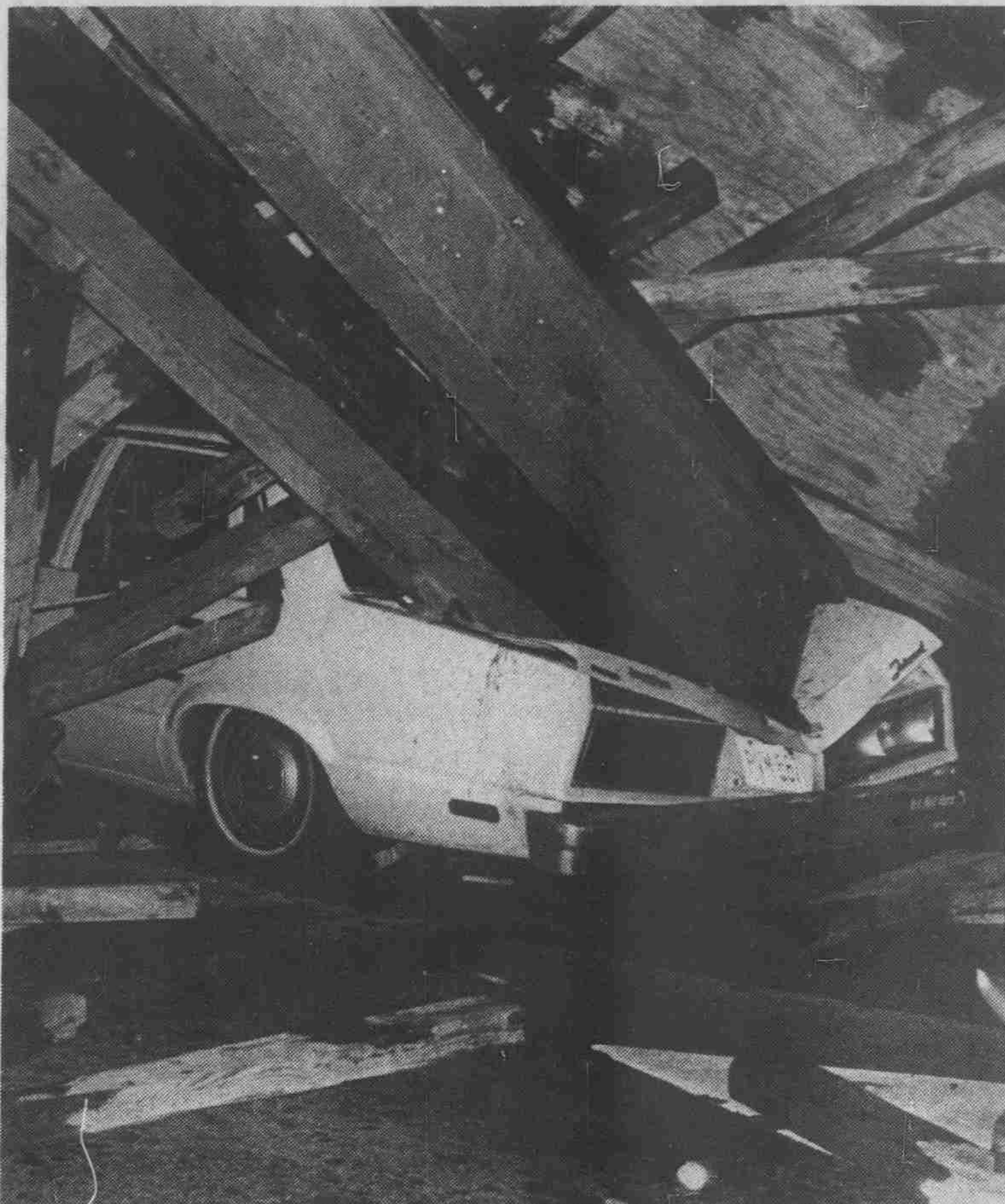
Road blocked, construction delayed, 'mega-buck' damage ...and it all happened on a Wednesday night
