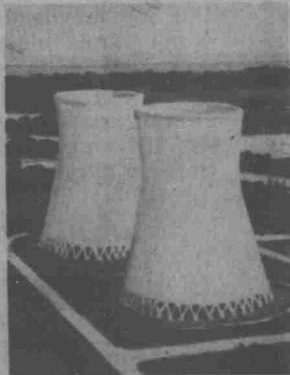
Cooling towers for reactor ...Maine plant stays open
