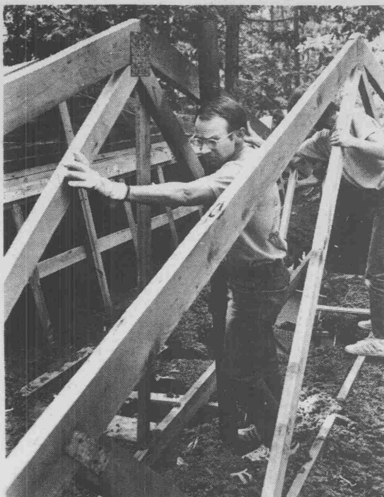
Neal Cheek of Habitat for Humanity removes roof frames from house.
