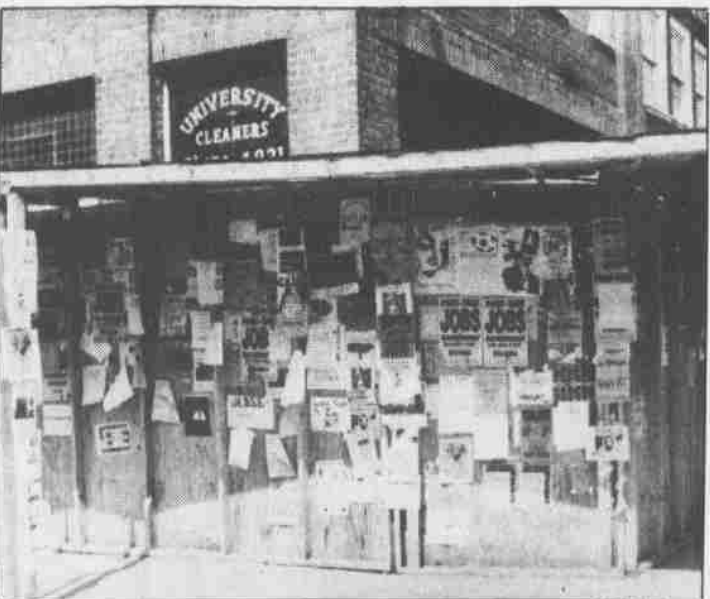
Hector's has remained closed from fire damage for six months
