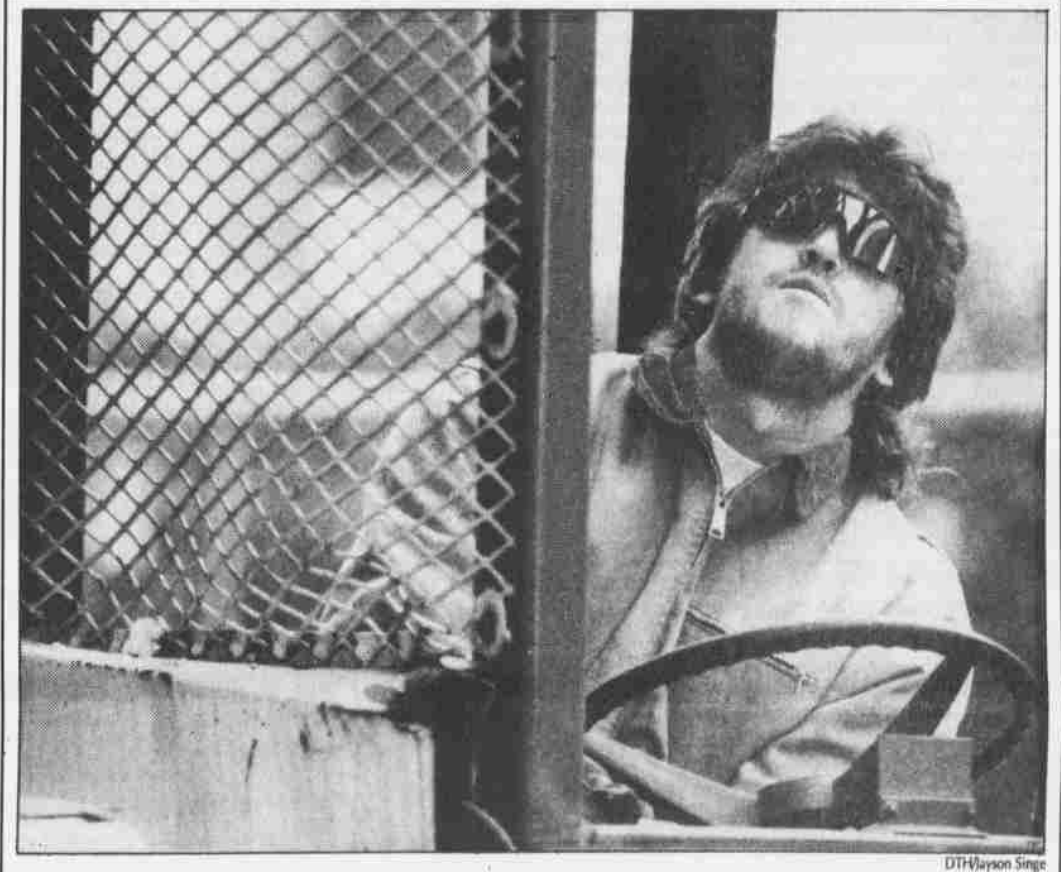
Workers began renovating the Student Union roof this week, destroying brick paths between the Union and Davis Library
