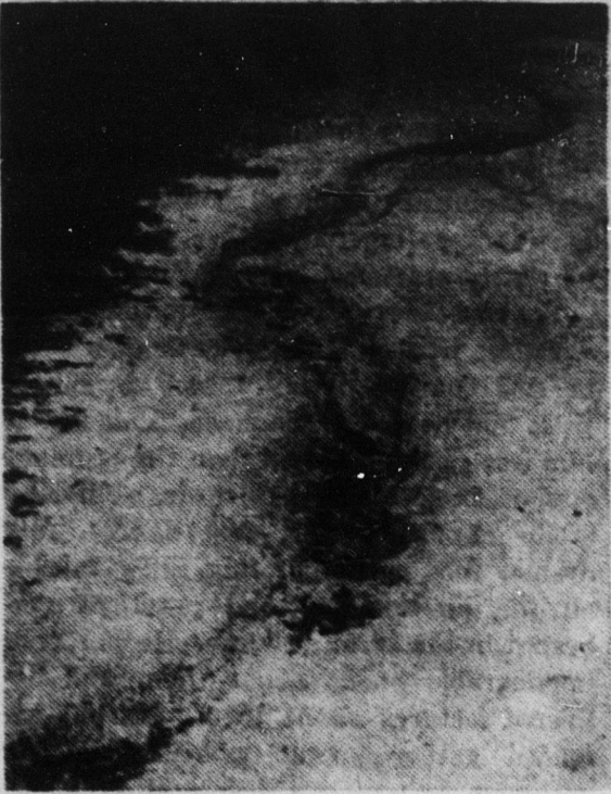
Here is one of the reasons why Chapel Hill needs brick sidewalks. This scene is on East Franklin street. Rains continue to wash dangerous gullies in the town's sand walks. Owners of 51 per cent of the property frontage on any given street may petition to have the town brick their sidewalk and charge them for the cost.
