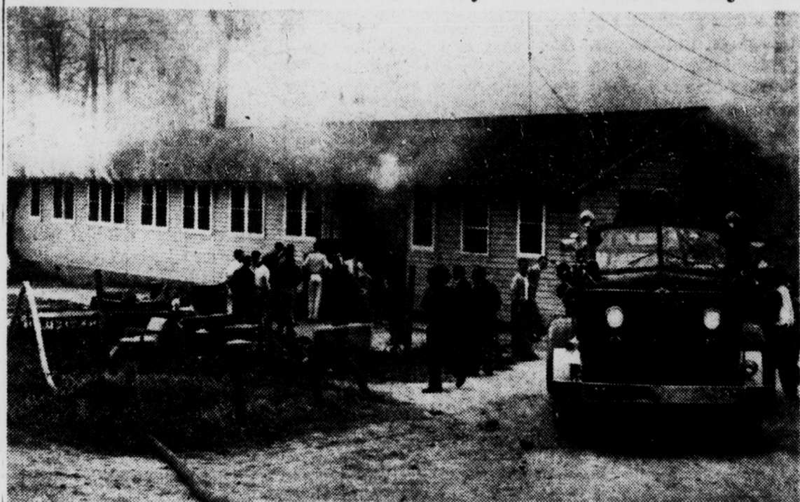
Here is the Victory Village Nursery, seen from Mason Farm Road, as the building burned Wednesday afternoon. Chapel Hill fire engine number three is to the right. The worst of the fire was centered in the kitchen and furnace room wing on the other side of the building.
