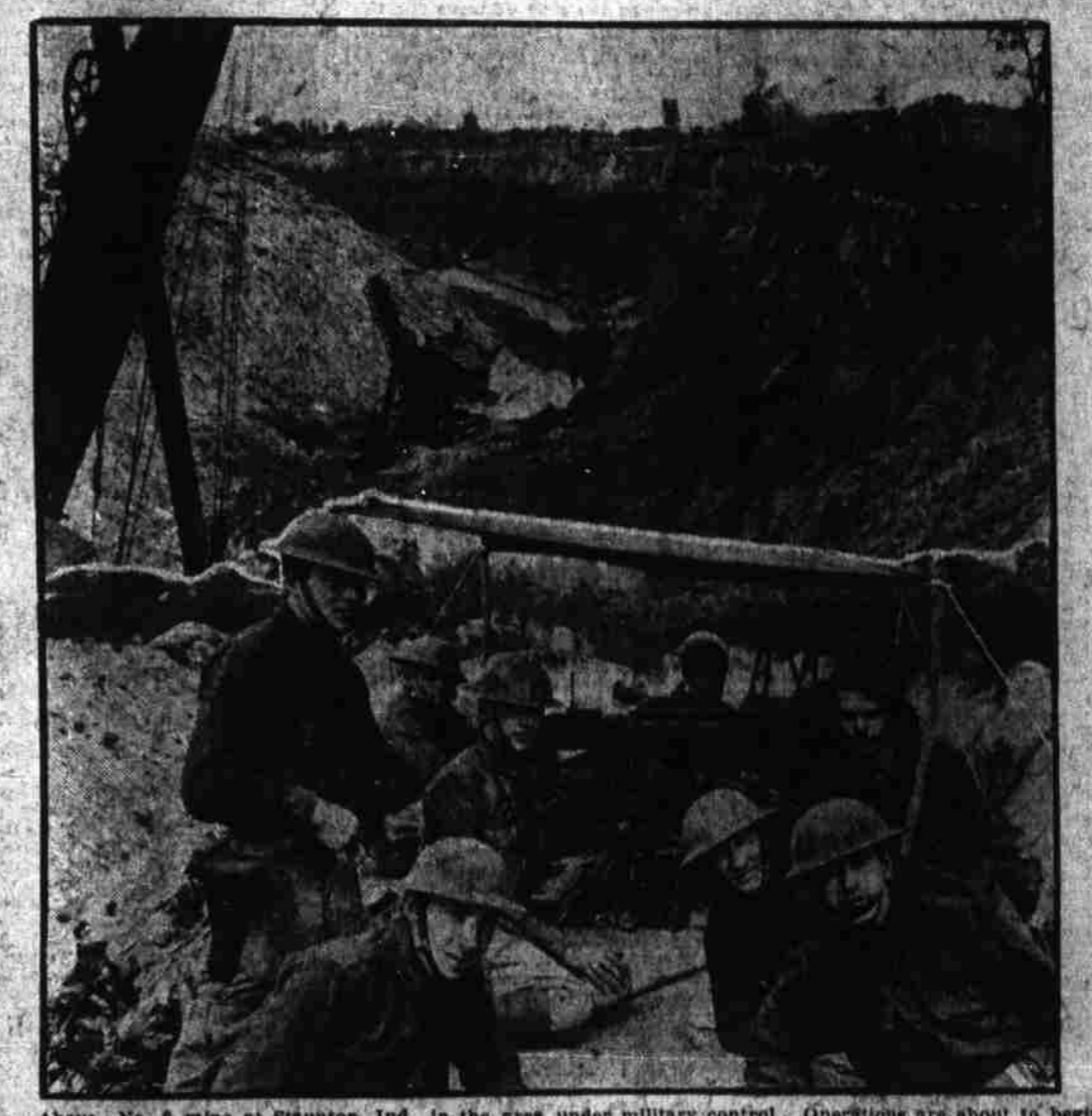
Above—No. 3 mine at Staunton, Ind., in the area under military control. Operations are about to begin in this area. The big steam shovel on the left is being closely guarded by details of state troops after reports were circulated that attempts would be made to wreck it. Below—Machine gun nest on a hill above No. 3 mine. Two men fired on a sentry guarding No. 3 mine from the woods in the background. This machine gun was used in replying to the sniper's fire. Indiana is mining coal in the strip pits near Staunton under a heavy guard of troopers. The Hoosier state is the first to take over actual production of coal in an effort to produce enough to supply the demand of state institutions and basic industries. The mining is being done under the direction of Governor McCray. Strike sympathizers made one attack on the guardmen, but were repulsed with machine gun fire. No one was wounded, say reports.
