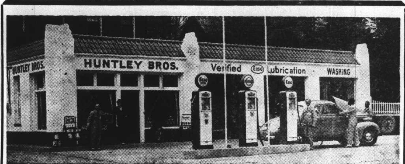
A View of our new Esso Station, complete and modern in every respect. We are prepared to serve you promptly and efficiently. Cars called for and delivered.
