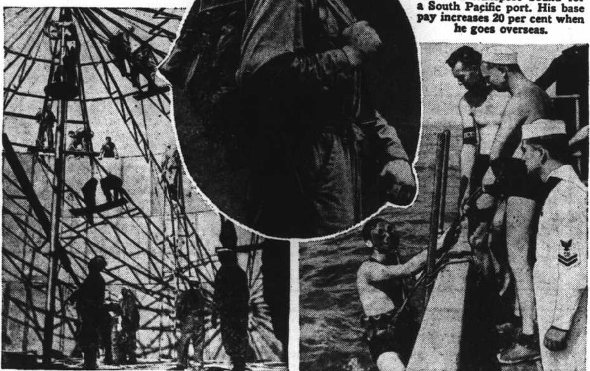
Constructing an oil storage tank. Fuel from this tank now supplies planes which are attacking Nipponese targets. In non-restricted manpower areas, men 18 to 38 may join by voluntary induction, while youths 17 and men 38-50 may enlist.
