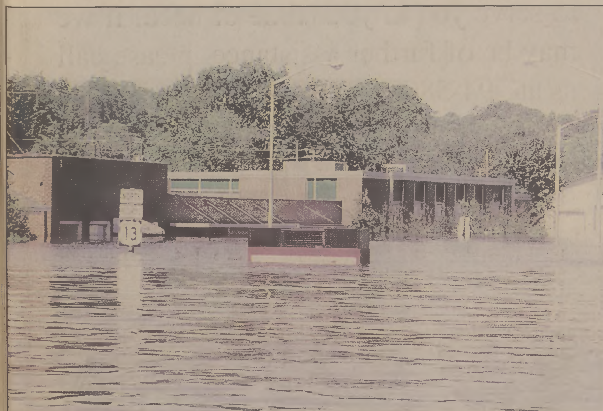
The record depth of the water on North King Street is evidenced by this Southern Bank sign, highway sign and the tops of the buildings. Eleanor's, Jake's and the U.S. Post Office are in the background. (Photo by Martha Price)
