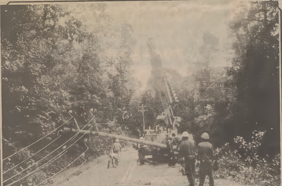
Flood waters, debris, and wind damage left from Hurricane Floyd makes restoration an unbalanced situation.
