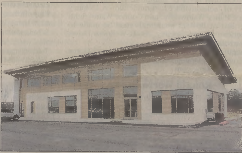
The new terminal at Tri-County Airport.
