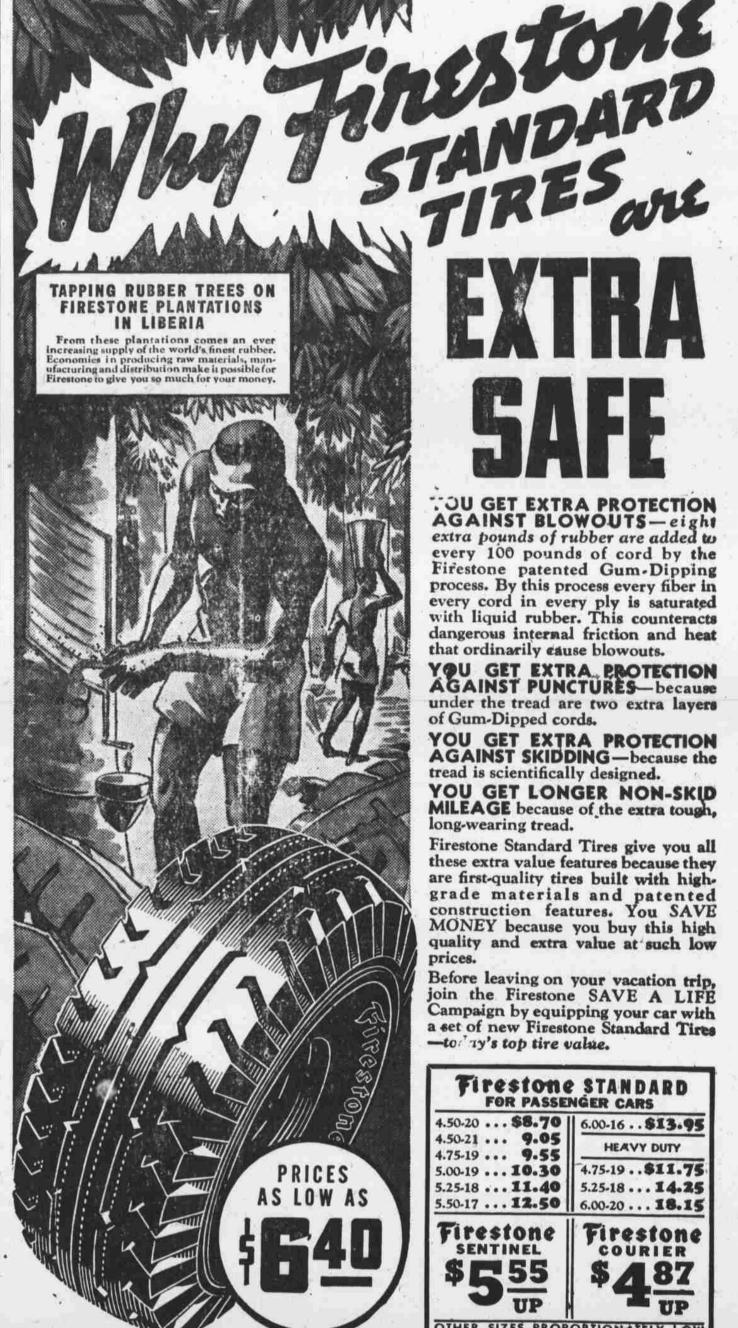
OU GET EXTRA PROTECTION AGAINST BLOWOUTS-eight extra pounds of rubber are added to every 100 pounds of cord by the Firestone patented Gum-Dipping process. By this process every fiber in every cord in every ply is saturated with liquid rubber. This counteracts dangerous internal friction and heat that ordinarily cause blowouts.
