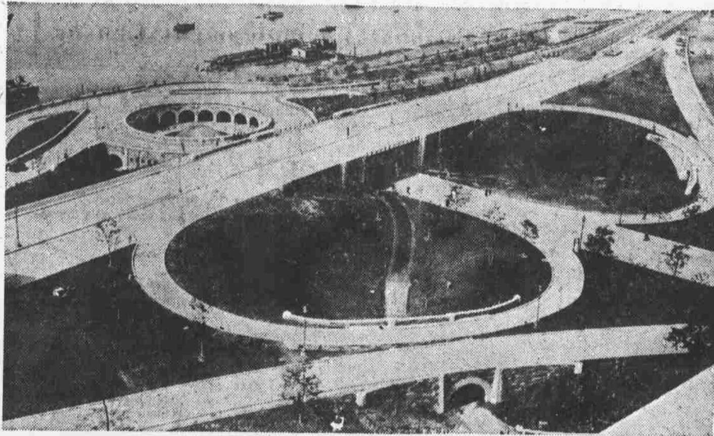
An elevation view of the traffic circle and fountain at Seventy-ninth street, New York city, showing part of the superhighway that is a big feature of the $24,000,000 improvement project on Manhattan's west side waterfront. Beneath this traffic circle is a garage accommodating 250 cars. A yacht basin and a promenade are other features yet to be completed.
