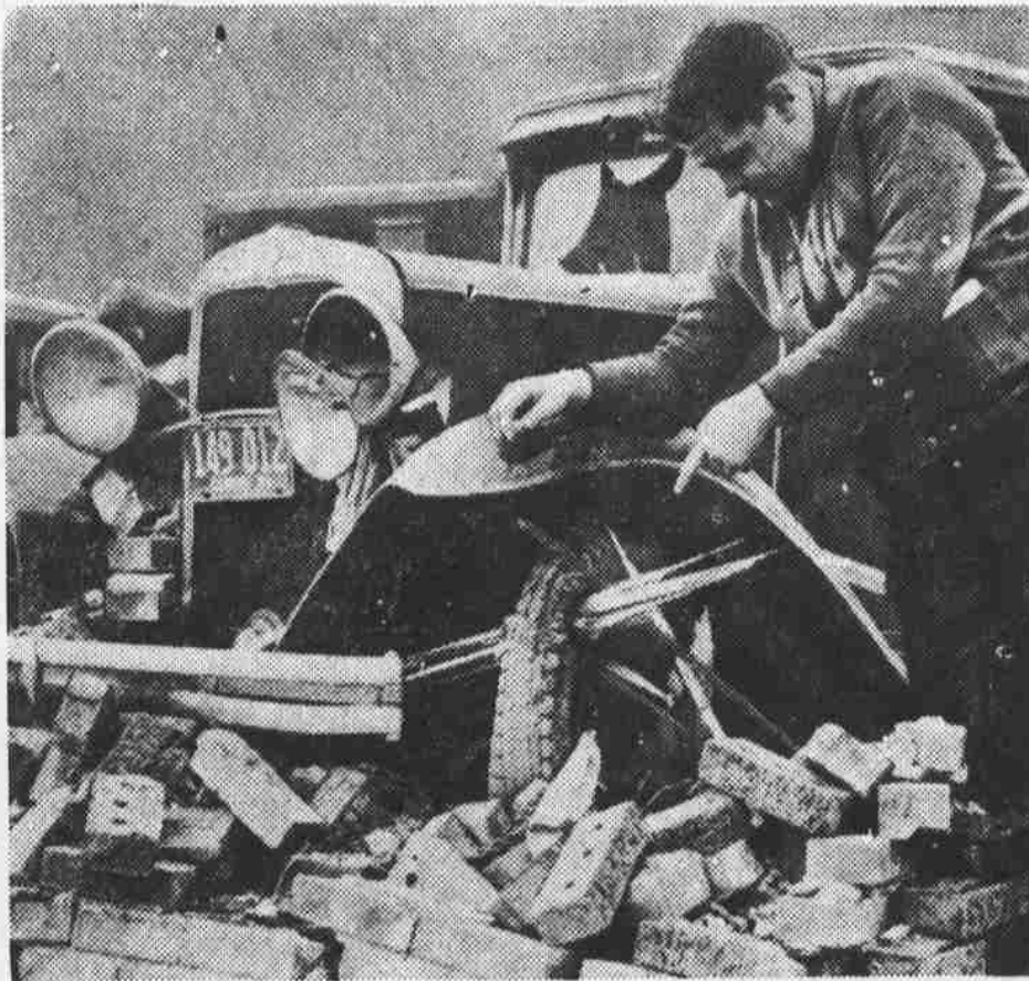
Property damage estimated at a million dollars and the loss of nine lives were the toll of a tornado that swept through Belleville, Ill., recently. This picture shows an automobile owner looking at his wrecked car. Note the piece of wood that went all the way through the tire.
