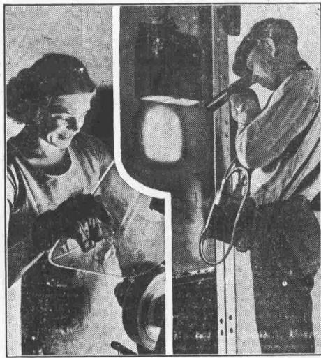
in automobiles. It is explained that one of the greatest hazards in auto acwas the most common cause of injury. girl at the left is polishing the rough Now all American cars are equipped edges of a car window.
