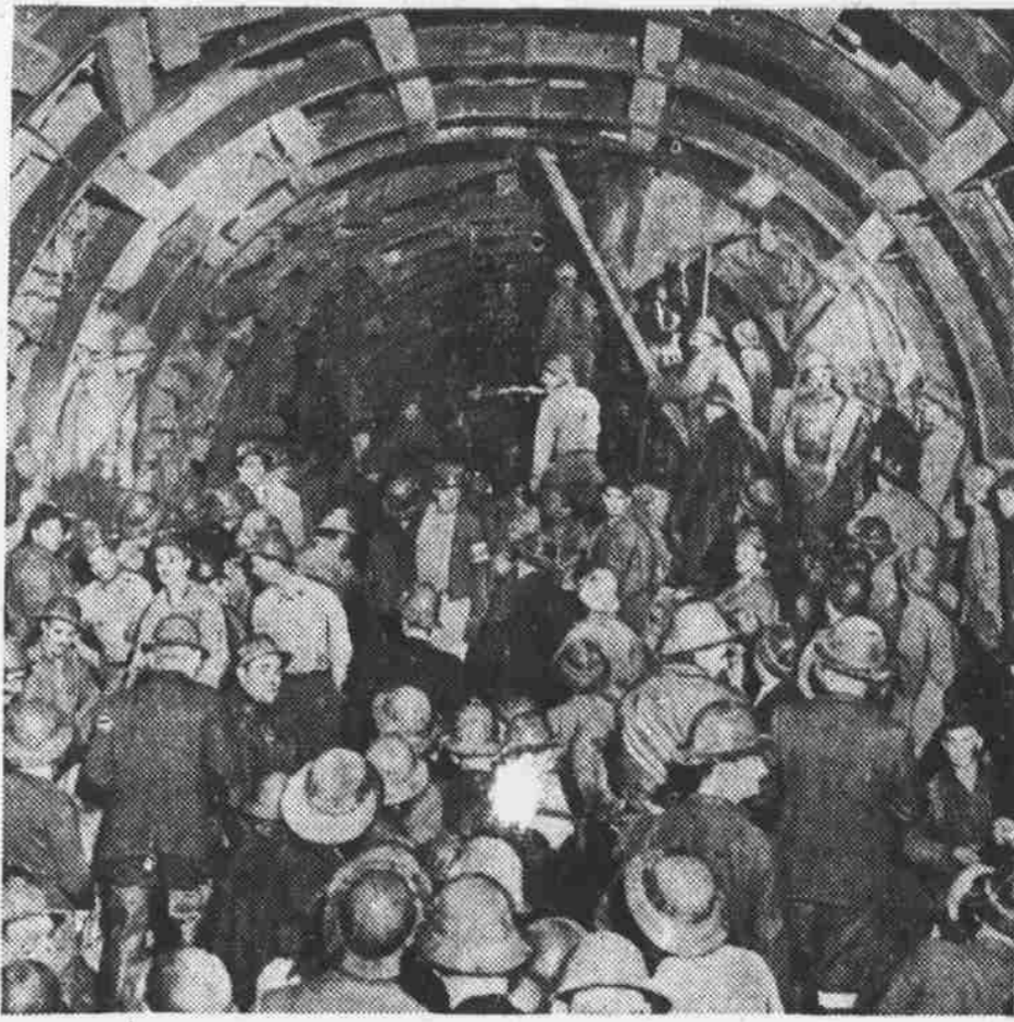
Completing a five-year job, hard-rock men holed through in the San Jacinto tunnel recently. Within a few months 1,000,000,000 gallons of the Colorado river will rush through this 13-mile bore daily in its haste to quench the thirst of Los Angeles and 12 other southern cities. It was one of the biggest tunneling jobs ever attempted.
