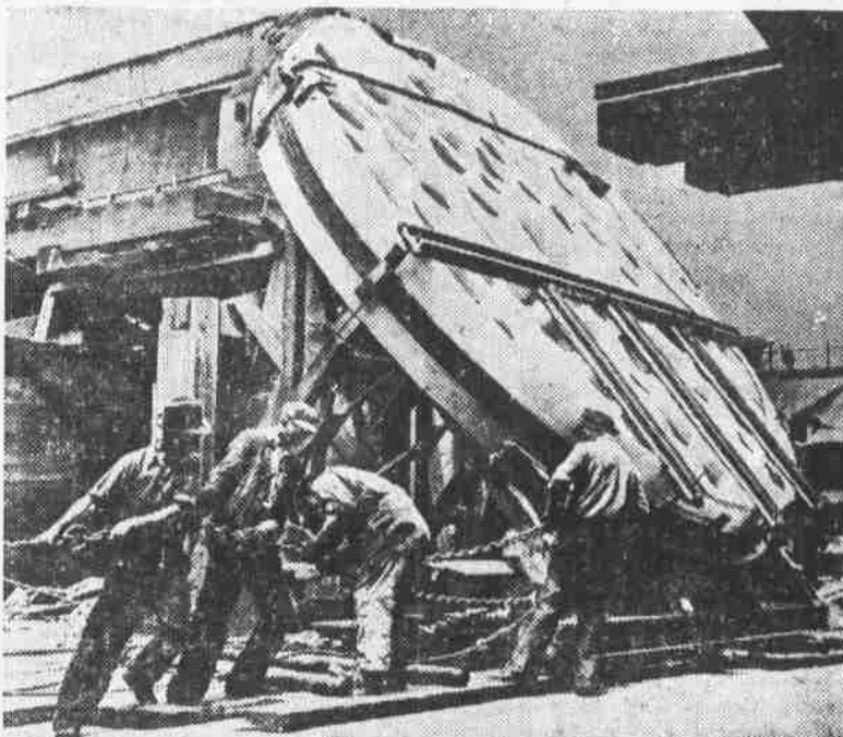
Using house-moving technique, workmen move the original 200-inch glass disc of a Corning, N. Y., glass works through a gap which was cut in a railroad trestle. An entire section of trestle and tracks had to be removed so that the huge 20-ton telescope eye and its special steel cradle could pass. The disc is the largest single piece of glass in the world.
