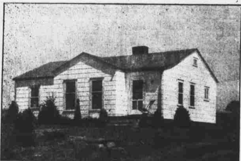
New home of Mr. and Mrs. Paul Carpenter on Whiteoak Street.
