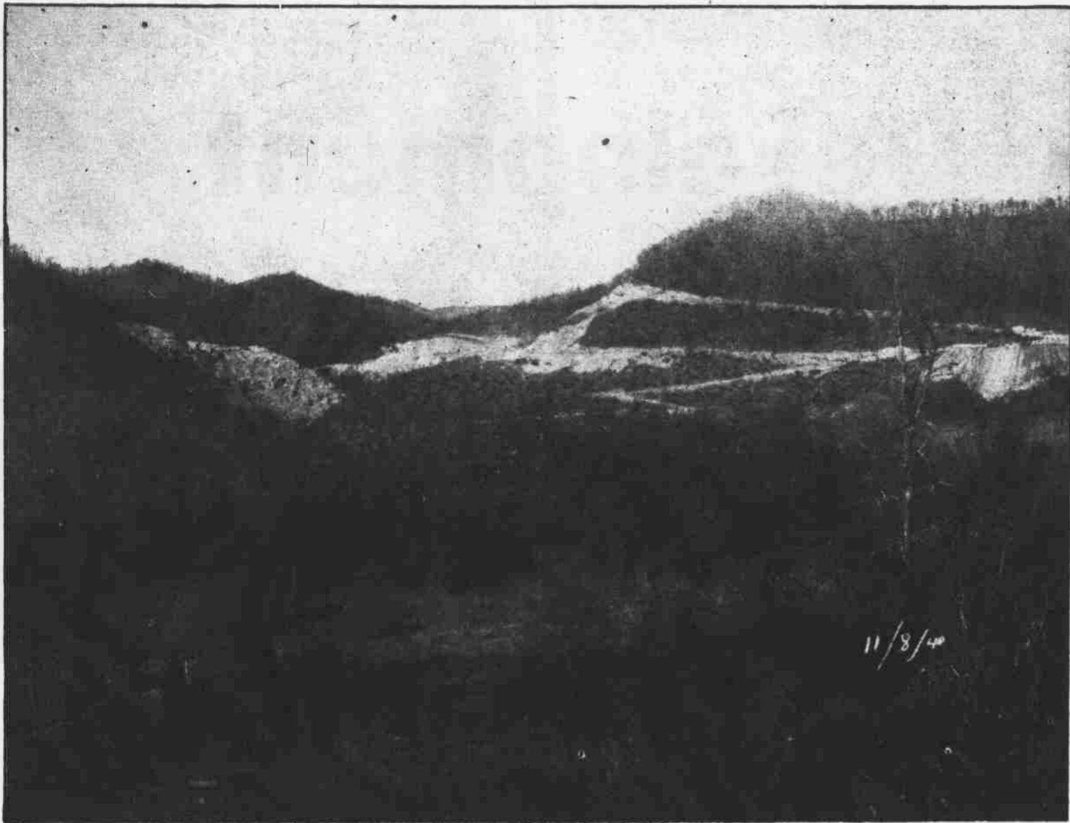
This picture was taken from a point on the Forest Service road between Kyle and the CCC camp near Aquone, looking down the Nantahala River. The left hand and right hand abutments of the dam may be seen.
