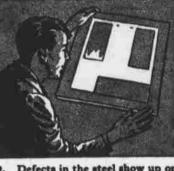
L. The new million volt X ray 2. Defects in the steel show up on built by General Electric saves X-ray film. Therefore faulty materials are tossed aside before costly hours of machining have been spent on them.
