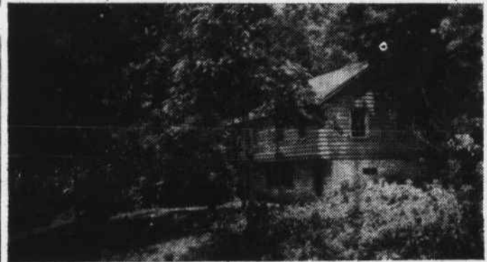
HERE'S COMMUNITY CENTER —Above is a view of the community house and health center at Nonah Center, on Cartoogechaye. The lower floor is used as a community gathering place, the upper will serve Cartoogechaye as a clinic.
