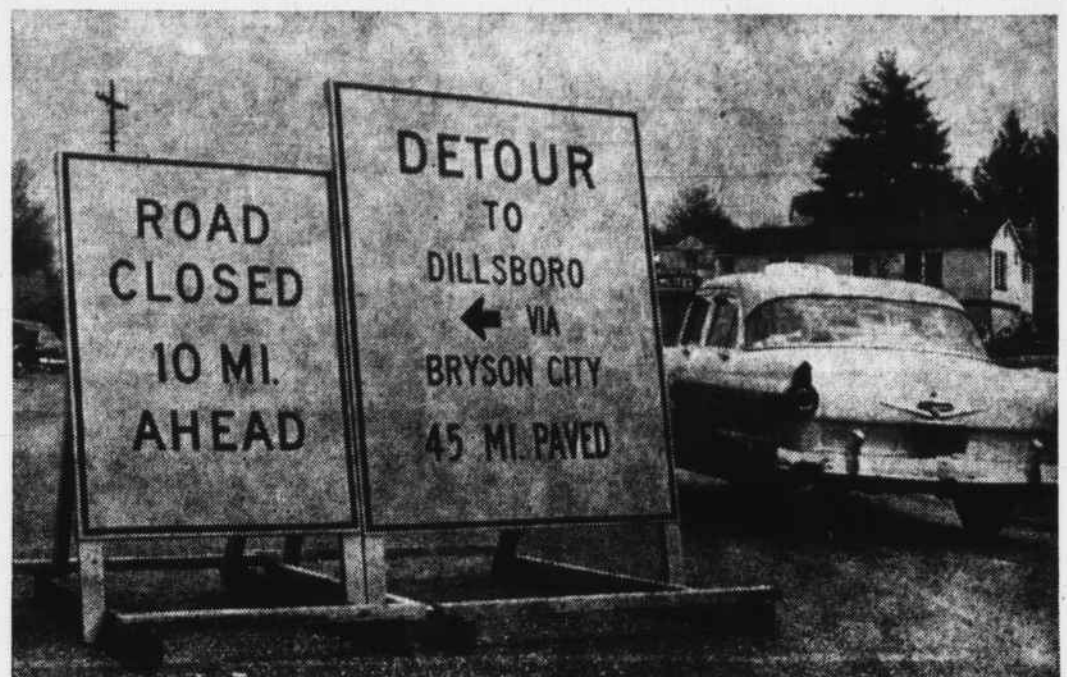
UP THEY WENT — Detour signs (not uncommon sights here in recent years) went up Tuesday on US 23-441 from Franklin to Dillsboro so maintenance crews could start repairing the damage to the highway caused by a large landslide two weeks ago. East-west traffic is being detoured through Bryson City. The job is expected to take about two weeks.
