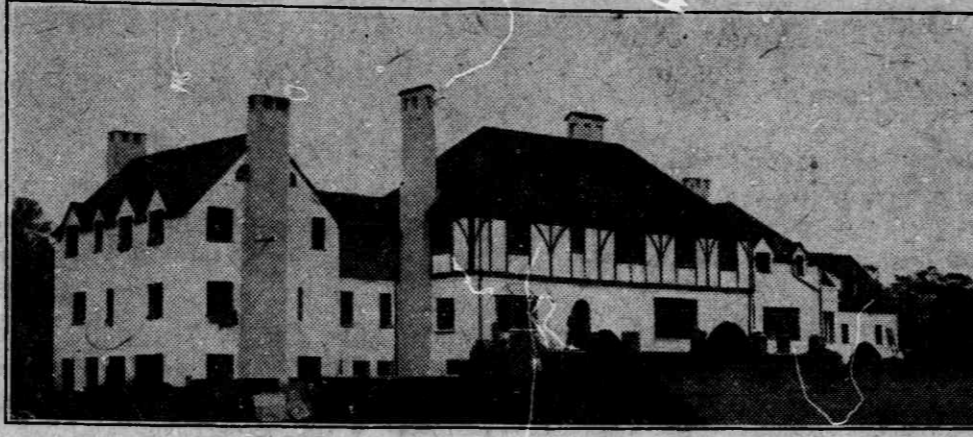
Residence of Mrs. J. A. Andrews, Now Nearing Completion on Site Overlooking Fort Bragg Country.
