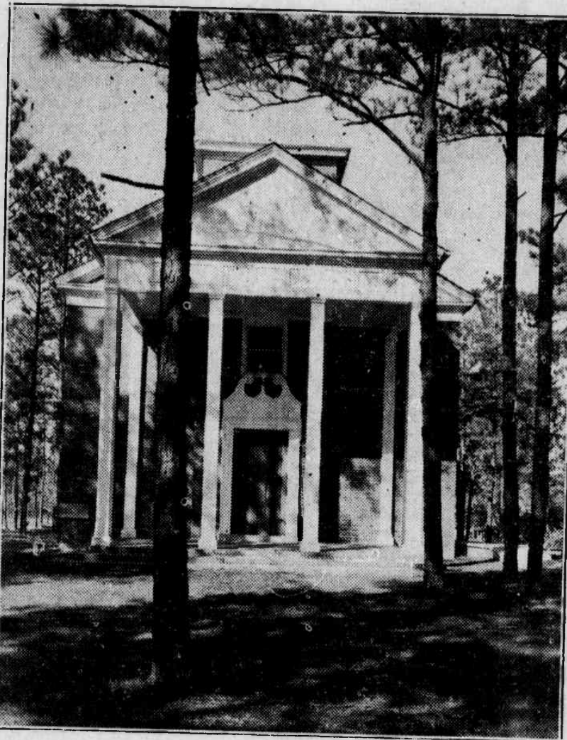
Presbyterians Turn Another Milestone In Their Meteoric Career in Southern Pines With Institution of New Heating Plant in May Street Edifice
