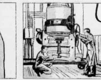
3. A regular check-up on pieces of 4. X-ray exposure needed for 5-X-ray film worn on workers' wrists inch-thick steel is now 2 minutes guard against prolonged instead of previous 31/2 hours! Whole days are saved in examinaexposure to the rays given off by tion of even thicker castings.
