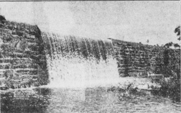
Top picture shows the huge expanse of water which now is backed up behind one new, steel-plated dam and a repaired old stone dam at Thagard's lake. The lower picture gives an idea of the spillway over the stone dam and also shows some of the leaks which John Warren Watson hopes will soon be plugged up, giving a two or three inch spill over the 40-foot spillway.
