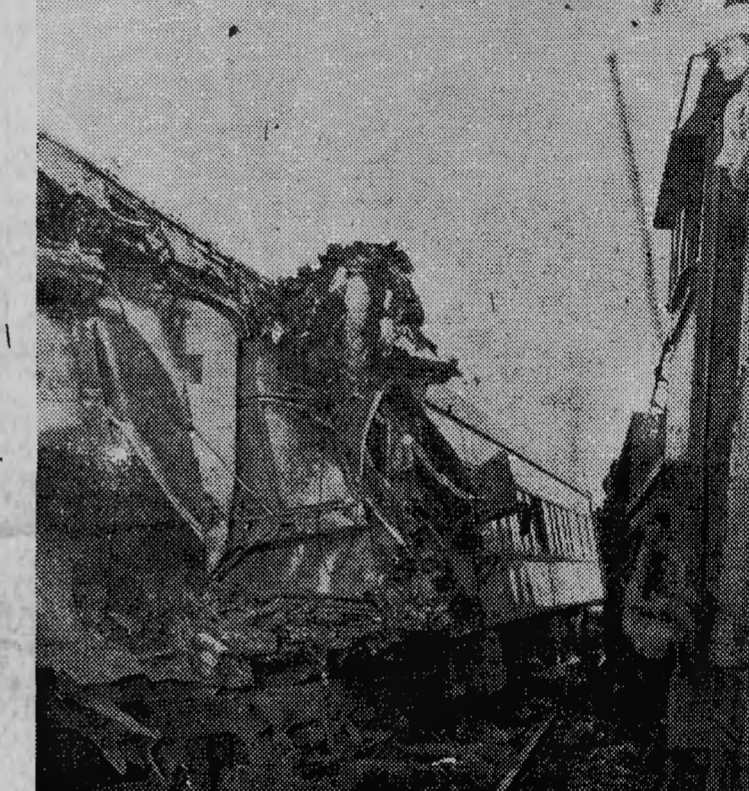
Pictured here are scenes of the Seaboard Air Line Railway wreck near Aberdeen early Saturday morning. In the upper picture railroad repair men are seen in center, repairing the track where the cars were derailed. In the picture below is a close-up of where the freight ripped the side of one of the passenger cars.
