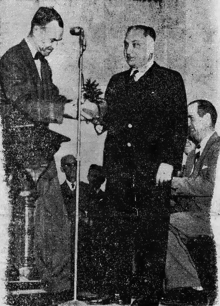
Top photo shows bulldozers and giant tractors breaking ground for the 4,000 square feet of floor space for the Carthage Fabrics Corporation. The plant is scheduled to be ready for occupancy by June, 1950. Lower photo shows Newland Phillips, left, secretary-treasurer of the investment corporation, presenting the first pot of earth from the site to Herman Chopak, chairman of the fabrics corporation and president of Chox K Fabrics, New York. State Senator W. H. Currie, master of ceremonies, is shown directly behind Chopak. (Photos by Staff Photographer R. W. Stephens.)
