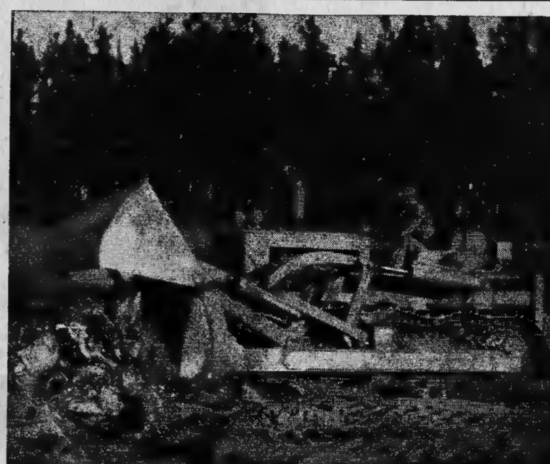
And Then Buried In Trench By 'Bull Clam'
