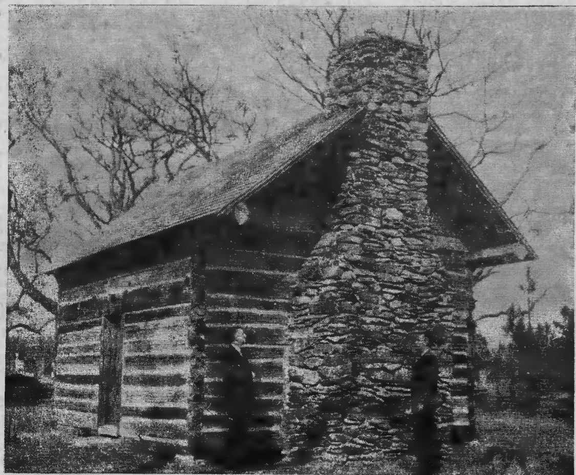
RESTORED CABIN —J. W. Causey, left, and Roy Newton, members of the Moore County Historical Association's restoration committee for the log cabin moved to the Shaw House grounds, are shown here inspecting the completed structure. They are looking at the chimney, built by Ed Calcutt who lives between Southern Pines and Aberdeen, with stones fitted together
