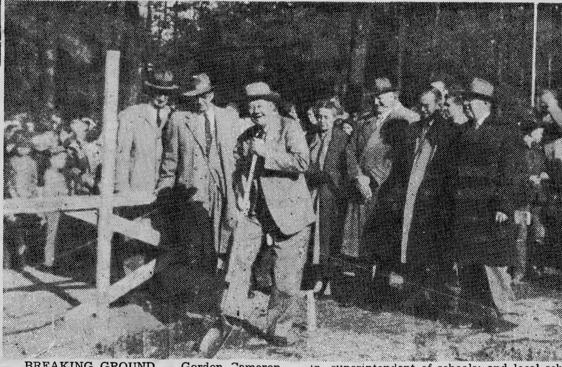
BREAKING GROUND — Gordon Cameron, chairman of the board of county commissioners who appropriate funds for school buildings, wields the shovel as ground was broken last week for the new Southern Pines High School building at May Street and Massachusetts Avenue. Watching, left to right, are: A. C. Dawson, Jr., superintendent of schools; and local school trustees, John Howarth, chairman; Dr. Vida McLeod, who turned the first shovel of earth, Harry Menzel, L. F. Garvin of Manly, and Norris L. Hodgkins, Sr. In the background are students who witnessed the ceremony. (Photo by V. Nicholson)
