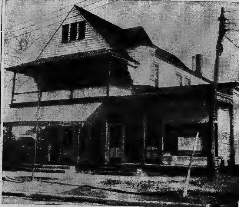
EVOKES MEMORIES —The former police station-ABC store building on New Hampshire Ave., is shown here as it looked when occupied. Owned by the town, it is now being razed and only the shell of the structure is standing. A town landmark, it once housed a pharmacy and physician's office and later a variety store. (Photo by V. Nicholson)
