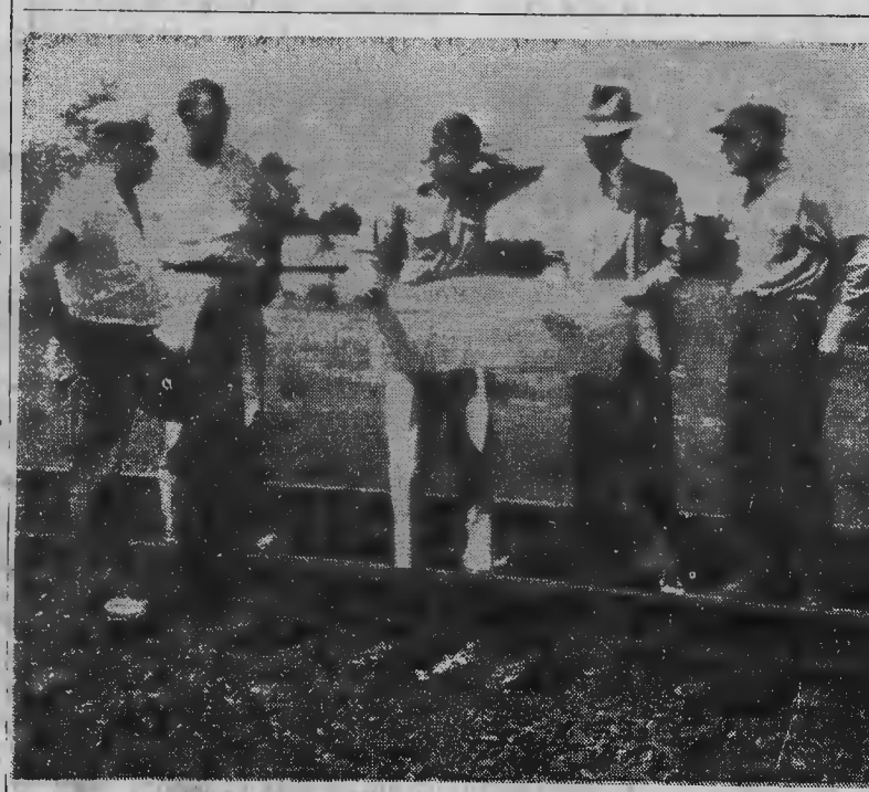
BY-PASS PLANNING—Seaboard Air Line Railroad and State Highway personnel are shown conferring at the site where the dual lane No. 1 highway by-pass will span the railroad on an overpass, between Manly and Niagara. They are deciding how railroad signal lines will be moved and protected during construction. Left to right: J. R. Power, Jr., Aberdeen, assistant signal maintenance, Seaboard; E. T. Powell, Seaboard signal department, Raleigh; Fred Beck, resident highway engineer, Carthage; C. B. Cole, Carthage, highway inspector; and H. J. Edge, Seaboard signal department, Aberdeen. Grading work on the by-pass route continued this week, with crews working north and south from the railroad bridge location. (Pilot Photo)
