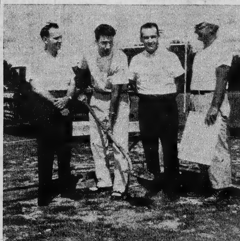
GROUND BREAKING for the new fieldhouse at Memorial Field was held last week with the four men above sharing the honors. At left is Bill Thomasson who has headed a drive to secure funds for construction of the building; next to him is Jim Walsler, the new football coach; third from left is Luther Adams, superintendent of the city school system; and at right is Burton Perham, contractor. Plans for the building were donated by Thomas T. Hayes local architect. Thomasson said he was looking for funds to complete the structure and suggested that 100 people willing to donate $10 each would do the trick. (Humphrey photo)
