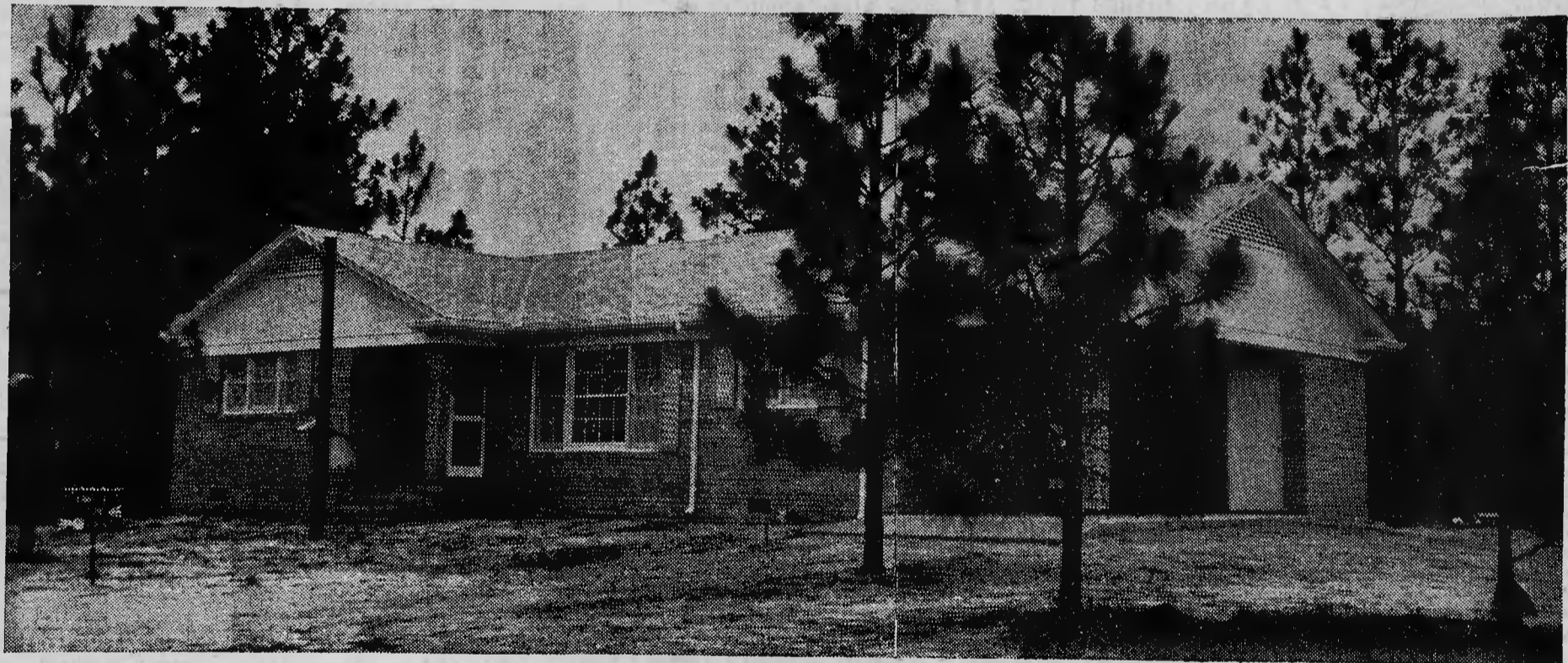
Medallion Home built by M. C. Almond—full HOUSEPOWER, wiring by Aberdeen Electric Shop.
