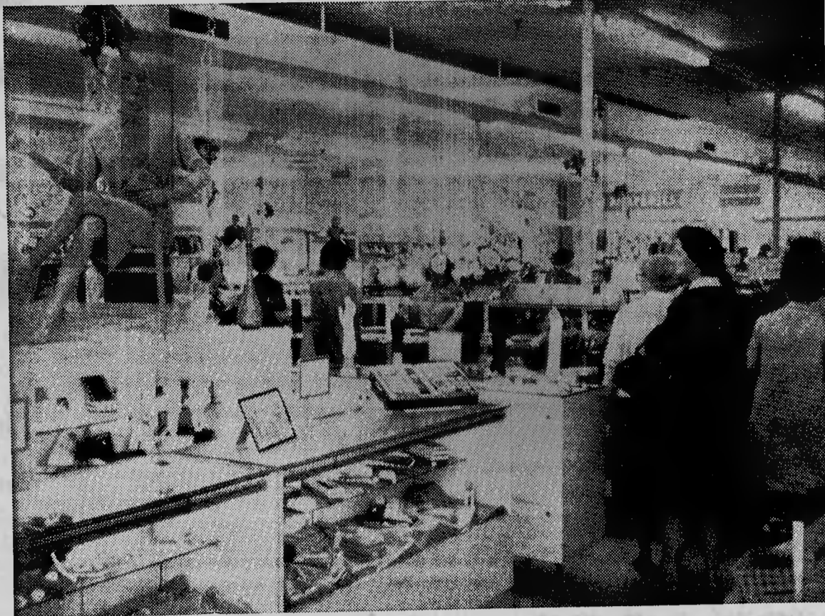
General View of Enlarged and Redecorated Store
