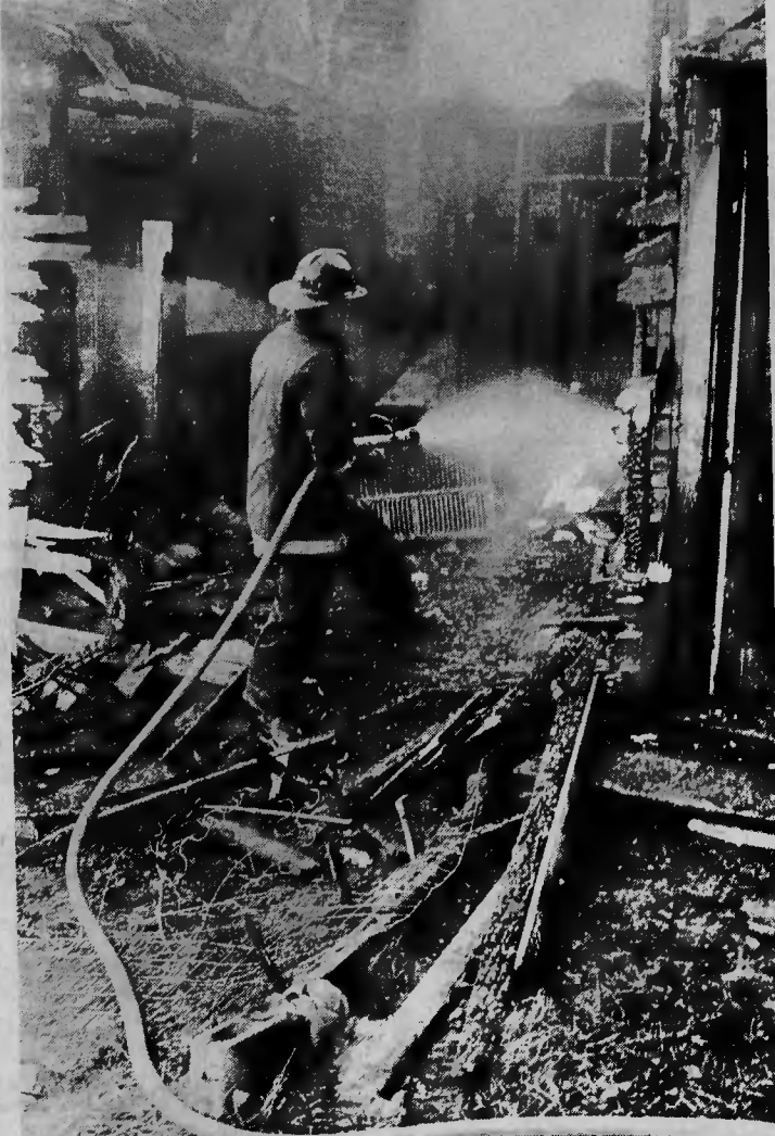
DESTROYED —This six room frame house belonging to Curtis Chavis was completely destroyed by fire Sunday afternoon. It is located on rural road 1897 near the airport, and both Whispering Pines and Carthage units responded to the call. Firemen spent almost three hours on the scene, and here one of them directs a stream of water into the living room area where the blaze is believed to have started. (Photo by Bryan Green).
