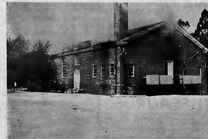
AT MIDDLE SCHOOL—Fire that broke out at Southern Pines Middle School around 10:40 today was immediately brought under control by Southern Pines firemen. The fire broke out in the auditorium and damaged the stage curtain, the Fire Department said. (Photo by V. Nicholson).
