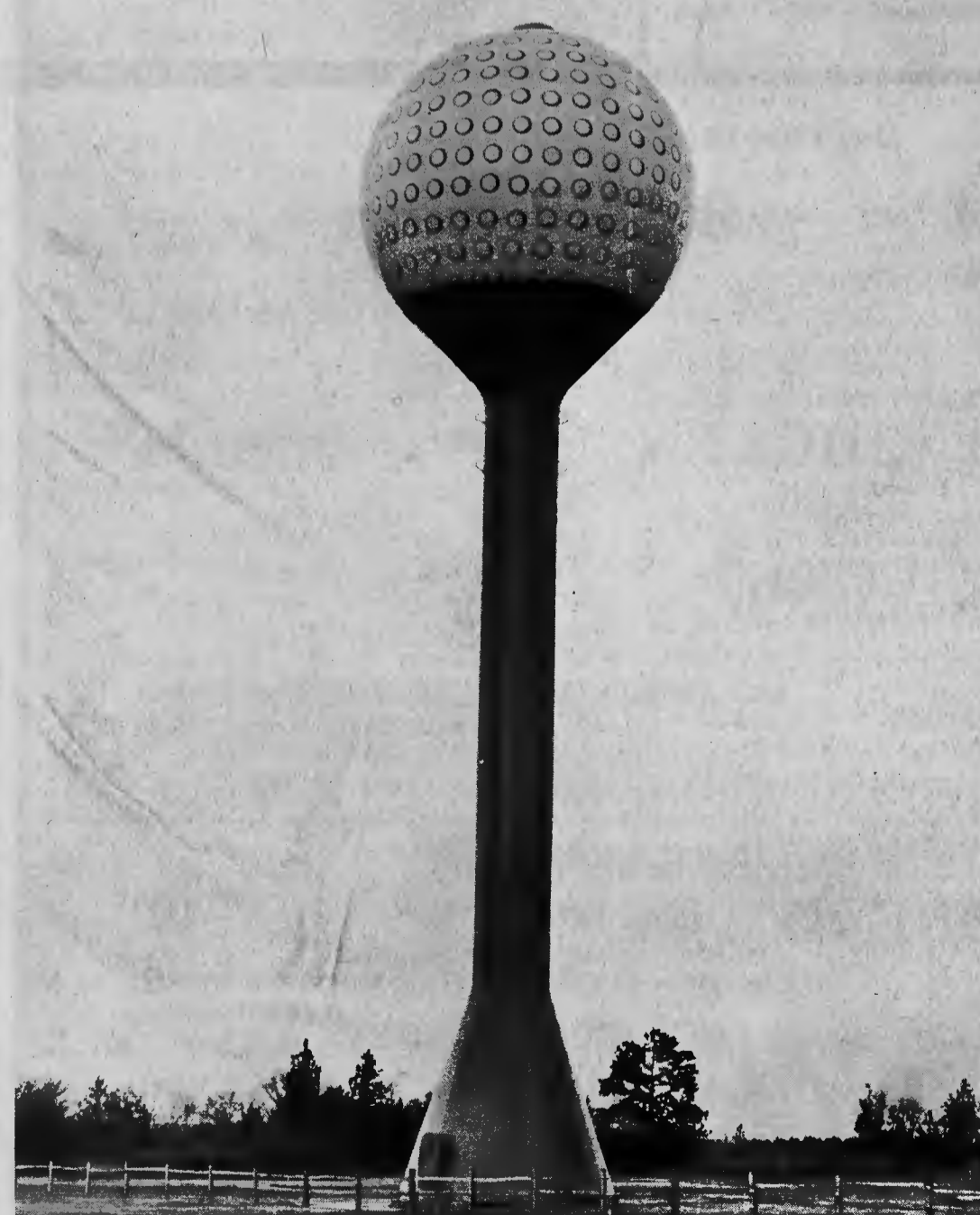
GOLF BALL — What is probably the largest golf ball in existence is this one at Seven Lakes. It is actually the 150,000 gallon water tank for the big new development near West End. (Photo by Alvin Davis).
